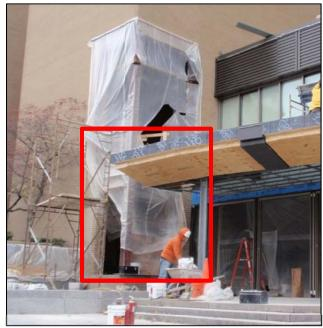
Figure 5 Opening Created for Micropile Drill Rig
