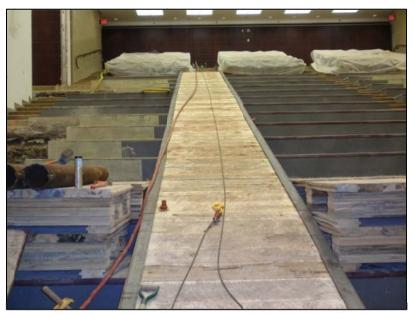
Figure 6 Track/Ramp used for Micropile Drill Rig
